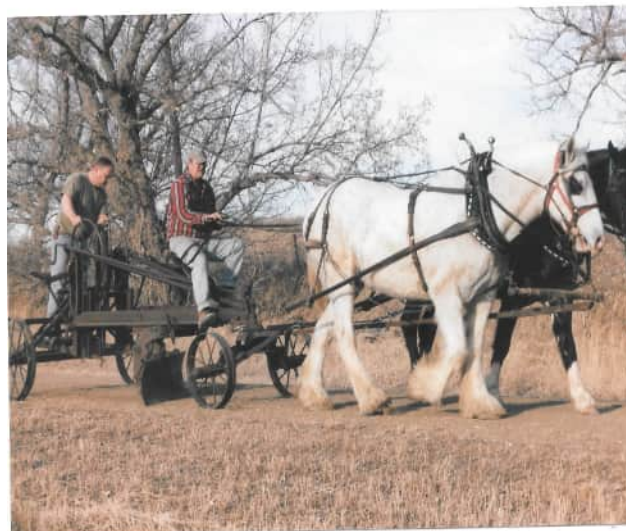
Glenn Zink is driving the team pulling the road grader used on Basin Township roads by his grandfather Royal Hawley Zink. Craig Zeisler is operating controls on the machine.
